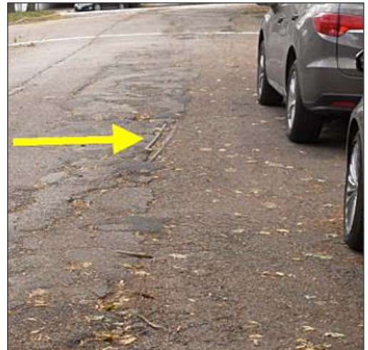
Rail Channel in Asphalt
